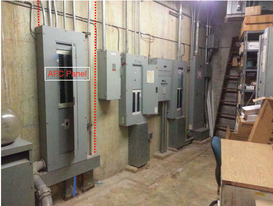
#AM2 Photo #5 – Existing and Proposed Route in Room C106
