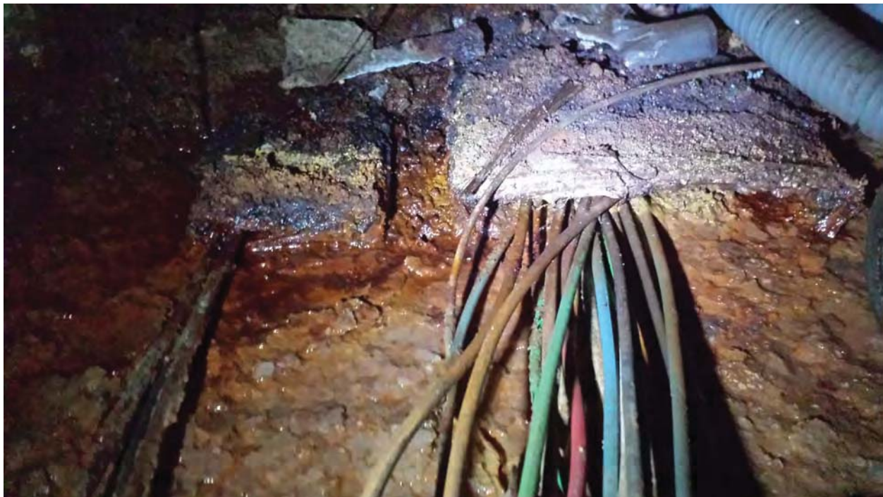
Photo #6 – Condition of Existing Duct inside Kiosk
